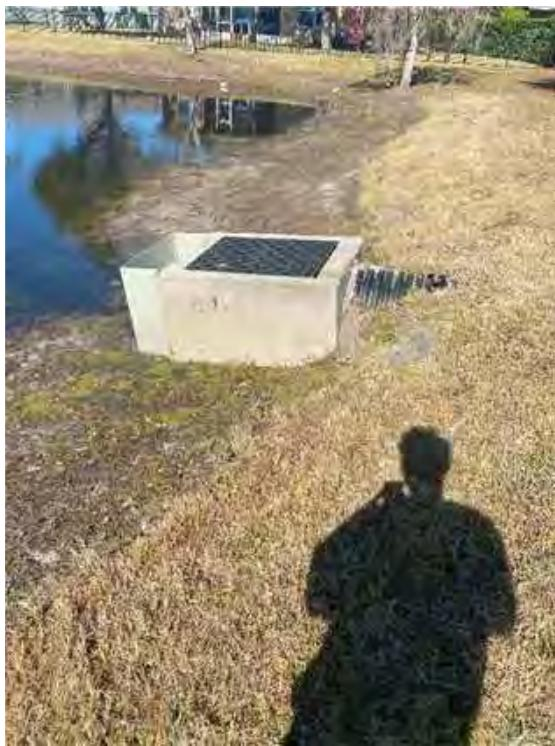
**Location 10:** Fence Down. To be reinstalled. Approach slab is undermined. Place fill, rip rap and filter fabric at approach and discharge slabs to deter future erosion. Fill voids with grout or compacted soil. Use outdoor grade sealant to seal the gap between the structure and approach slab to deter water intrusion and undermining. Remove vegetation from structure.
