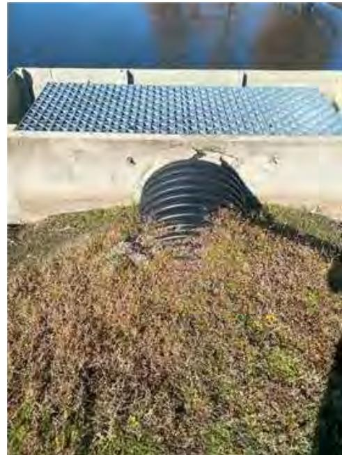
**Location 3:** Clear overgrown vegetation 5' around outfall structure and cover exposed pipe with filter fabric and fleximat and sod all disturbed areas.
