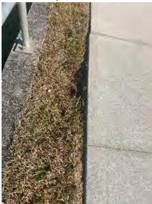
**Location 2:** Clear overgrown vegetation 5' around outfall structure and cover exposed pipe with filter fabric and fleximat and sod all disturbed areas.
