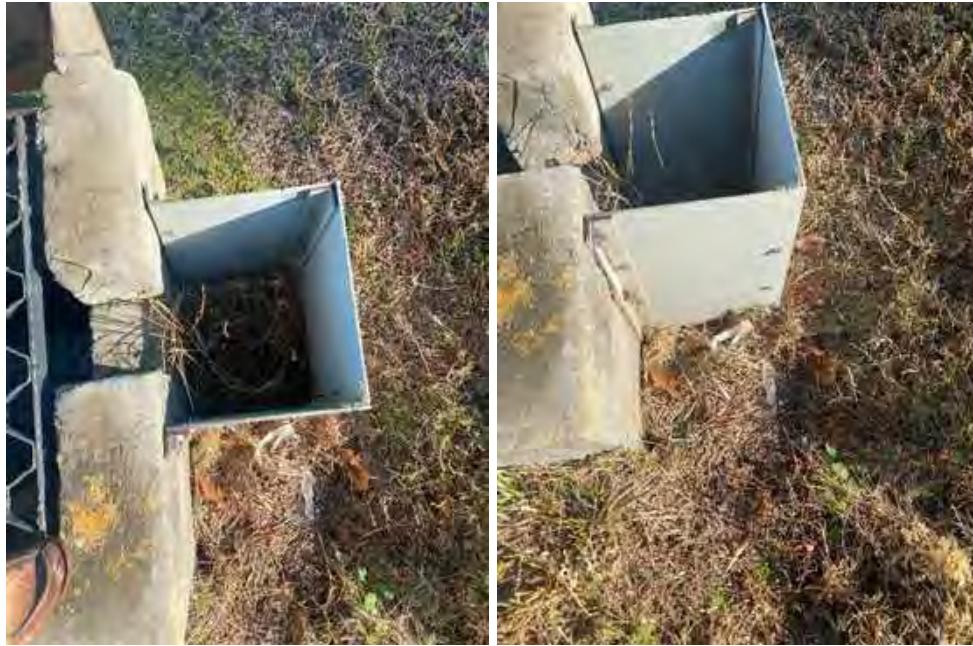
**Location 2:** Clear overgrown vegetation 5' around outfall structure and fix cracked structure. Grout inside and outside of structure for watertight seal.
