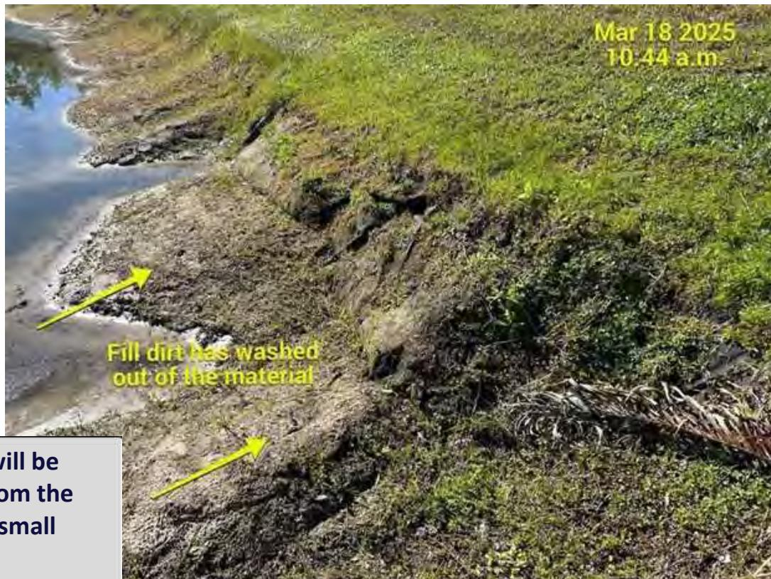
**The fill dirt will be recovered from the pond with a small excavator.**
