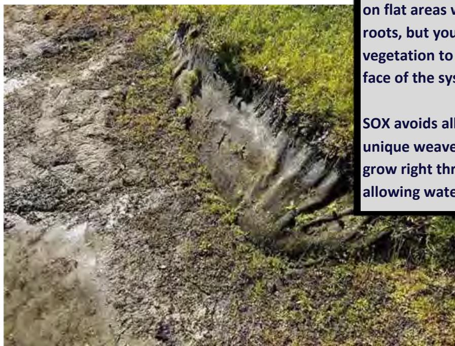
Non-woven filter fabric does not have the load bearing strength to support this amount of fill, especially heavily saturated fill after it rains.
