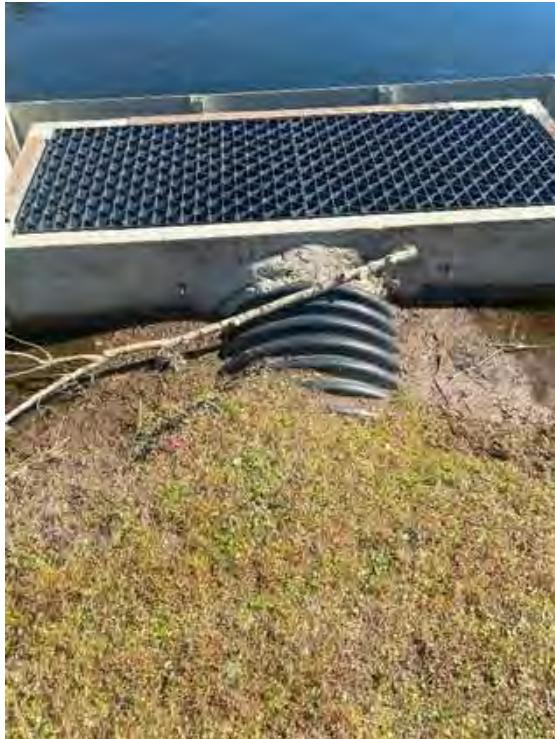
**Location 8:** Clear overgrown vegetation 5' around outfall structure and cover exposed pipe with filter fabric and fleximat and sod all disturbed areas.
